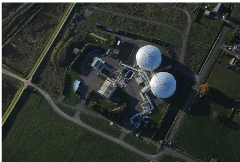
Hastings Waste Water Plant
